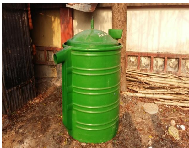
Installation of Kitchen waste processing unit nearby Canteen of main campus of Calicut, CMFRI for biogas generation for cooking on 31.10.16
