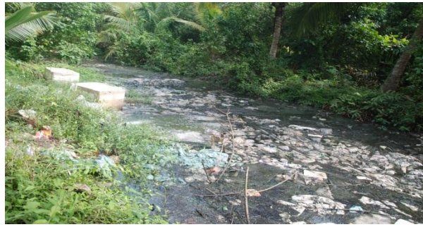
Canals clogged with litter
